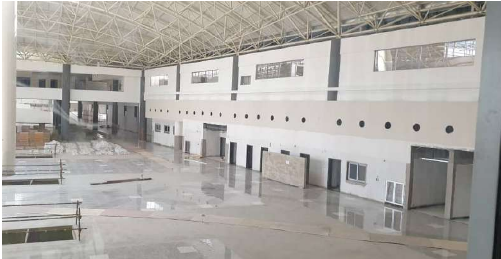
Inside of the Terminal Building
