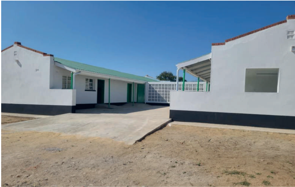
Umlugulu Clinic, Matobo RDC, Matabeleland South
