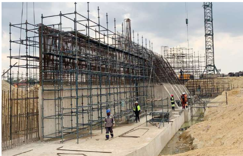
Mbudzi Interchange Construction
