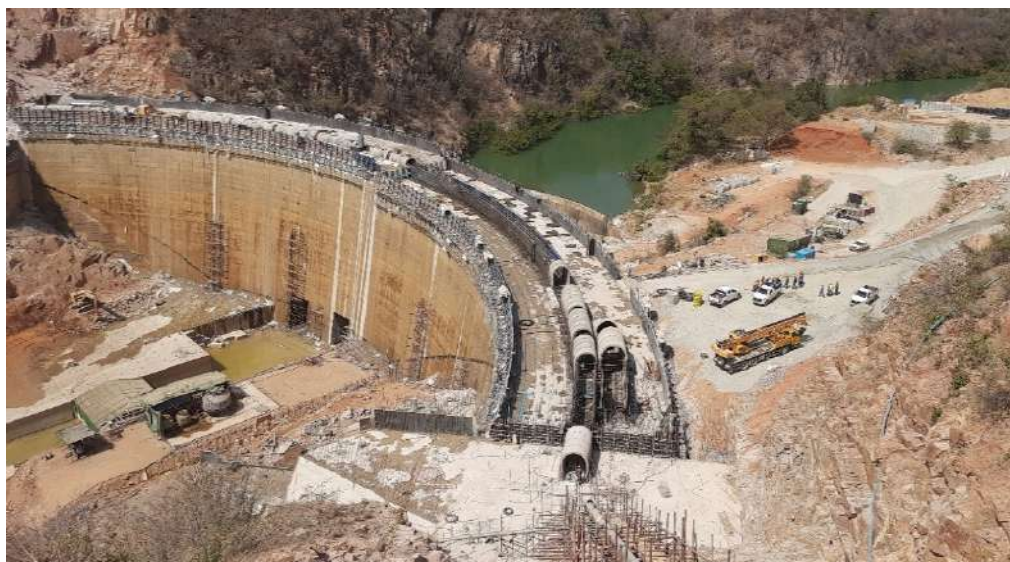
Gwayi Shangani Dam
