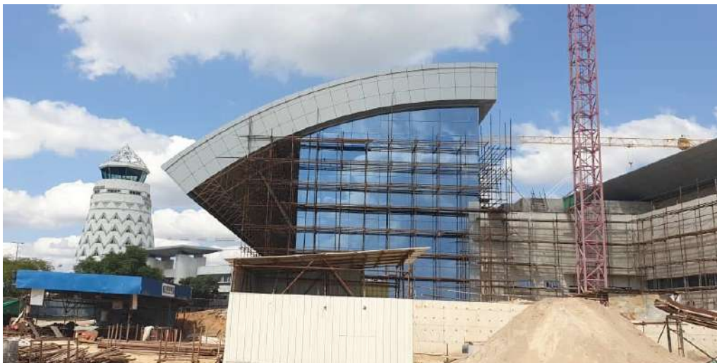
Outside of the Terminal Building
