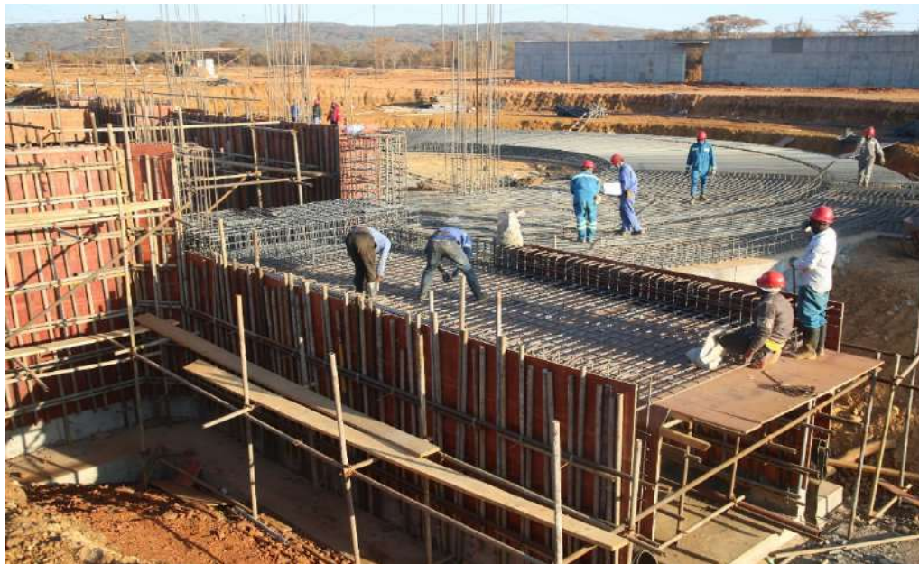
Construction at Manhize
